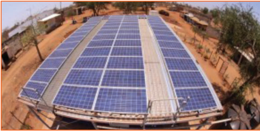
Fig.1 - Bird's eye view of the Trading Centre, solar PV canopy and the water tank. Two containers underneath the canopy hold the batteries and the system's switch gear and protection. One of the containers is used as the cooperative office.
