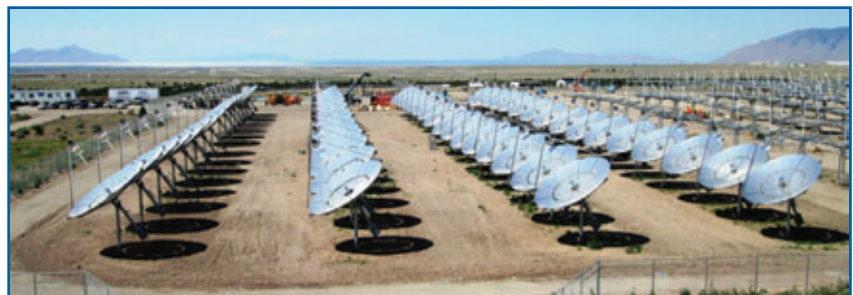
The Department of Defense’s presence in the western states is significant, and the military has continued to push the envelope on promising new energy technologies. This Stirling engine solar thermal installation (1.5 MWs) has just been installed at the Tooele Army Depot in Utah’s Tooele County.
