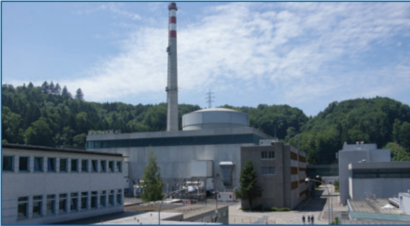
Fig. 1: Opened in 1972, the nuclear power plant in Mühleberg will be closed in 2019
