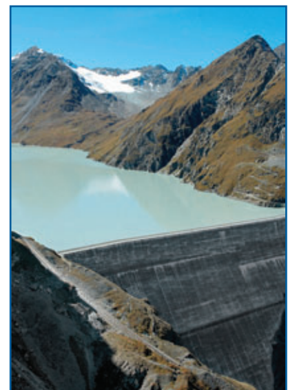
Fig. 2: At 285 metres, the Grande Dixence in the Swiss Alps is the world's highest gravity dam
